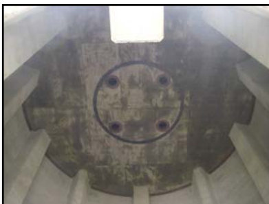
Finished elevated overhead slab
