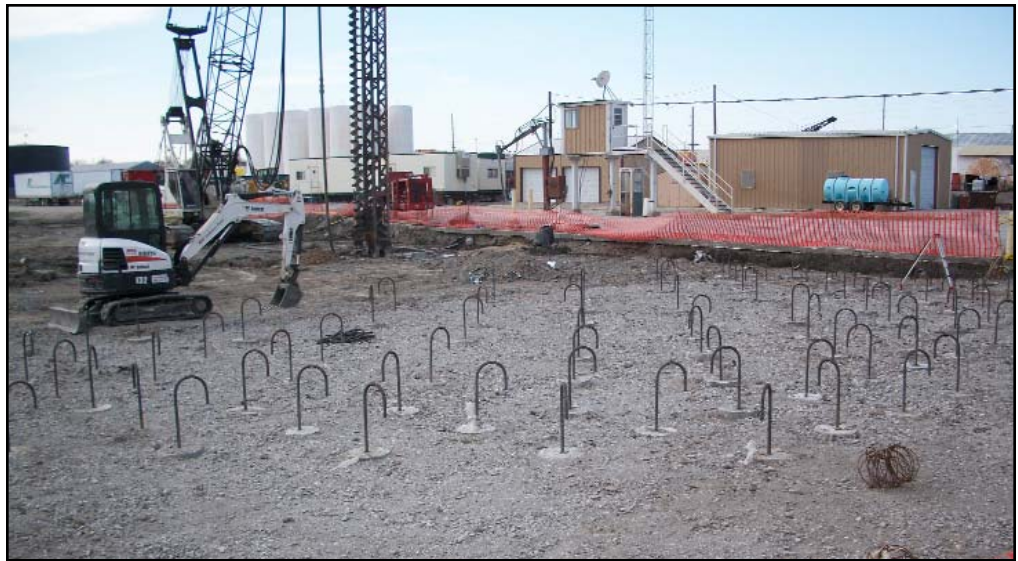
Installation of auger-cast piling
