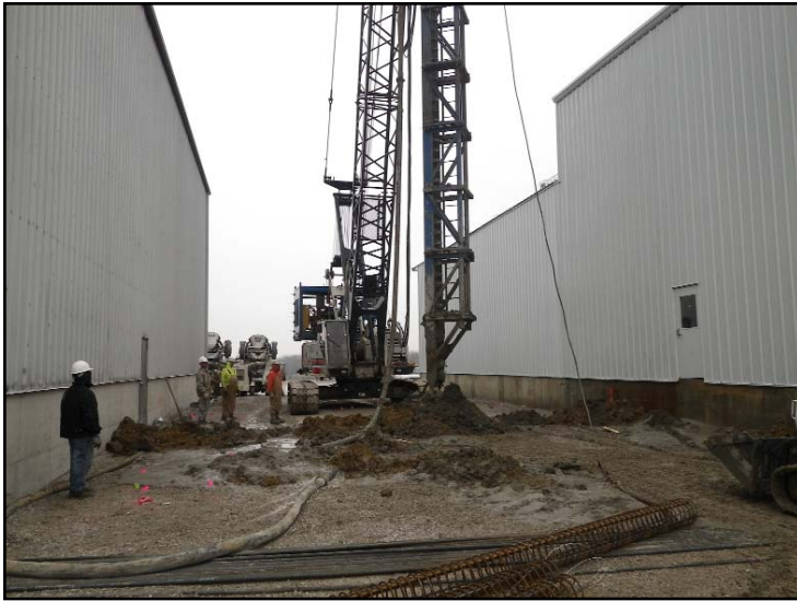
Installation of auger-cast piling
