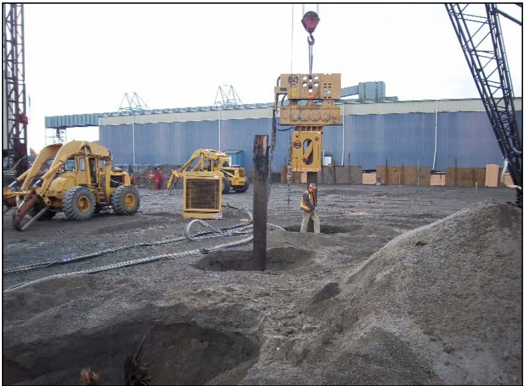
Existing structure deep foundation demolition (wood piling removal)
