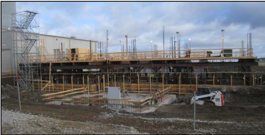
Slip forms almost ready
