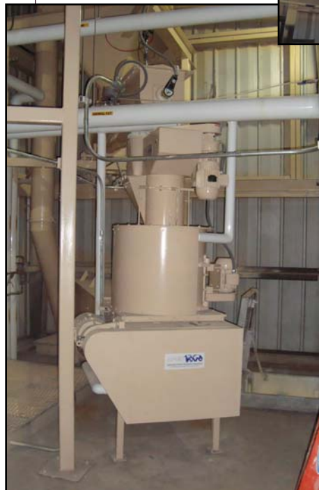
Above: Coater surge/weigh screw and fat delivery system
