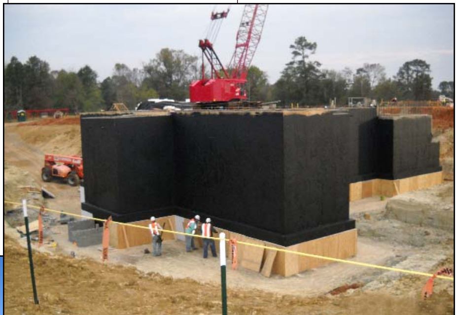
Above: Tunnel walls, waterproofed and ready for backfill
