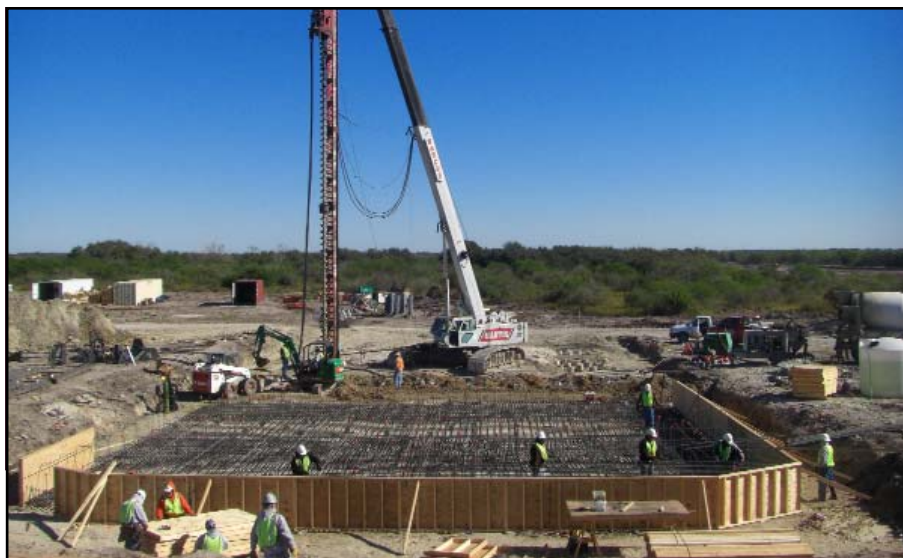
Placing auger-cast piling and mat slab form work and installing mat rebar
