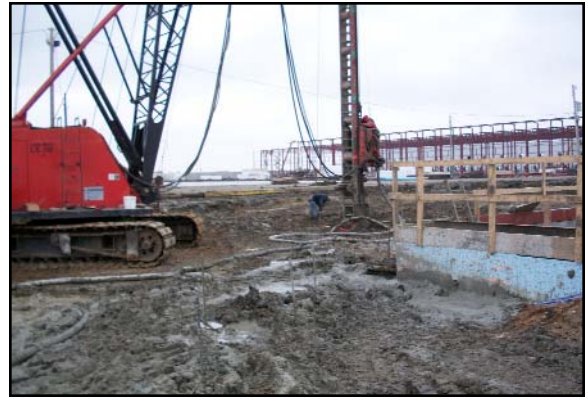
Drilling eighty-two 16"-diameter auger-cast piles
