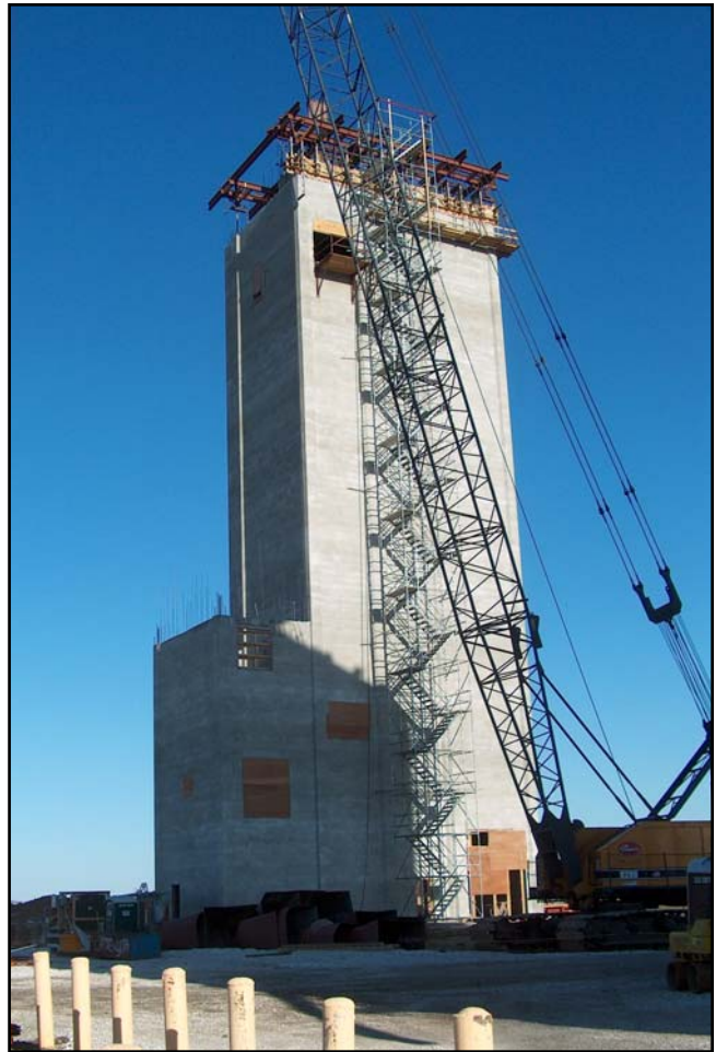
Wrecking off the slip forms
